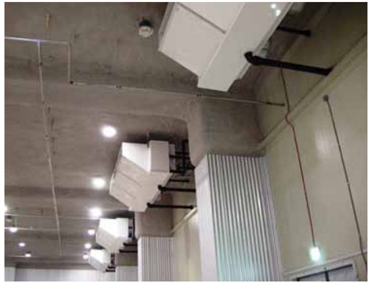
Equipped with diffusers, 184 Alfa Laval Helpman blow-through unit coolers can deliver regulated air-flow up to 65 metres, ensuring consistent temperatures throughout the Hyundai Logistics Osan Center, despite its size.
