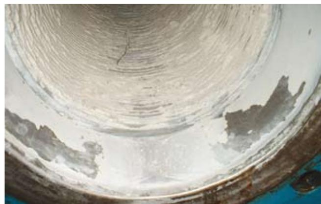
*Crystallisation of fluids when they get in contact with oxygen can deform and damage the plates.*
