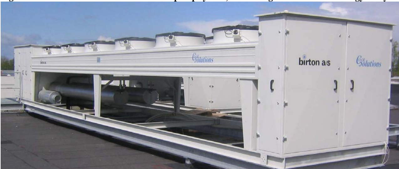
Figure 1: Outdoor unit with Birton thermal pump system, circulating CO2 with "free energy" only.
